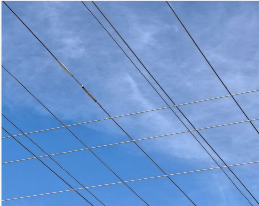
Photo 4: Conductor splices
