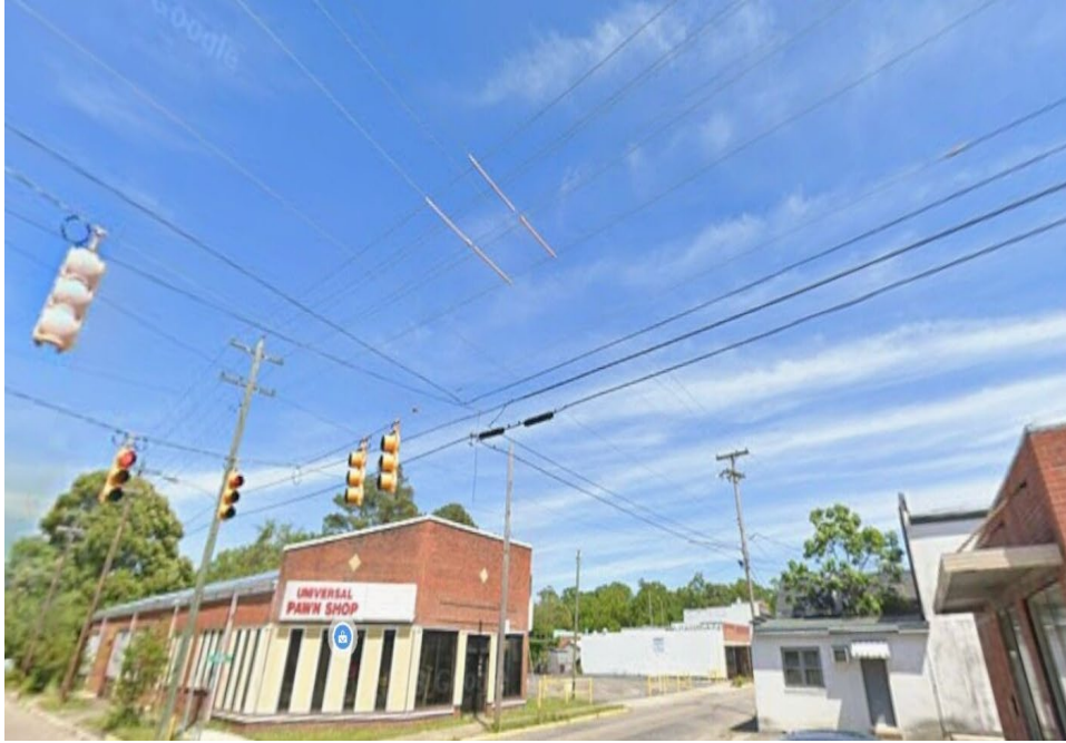
Photo 2: Line crossing prior to additional line spacing
